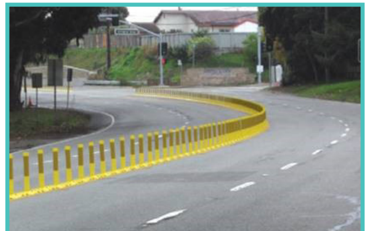
An example of the type of traffic separator that ODOT will install on OR 224.
