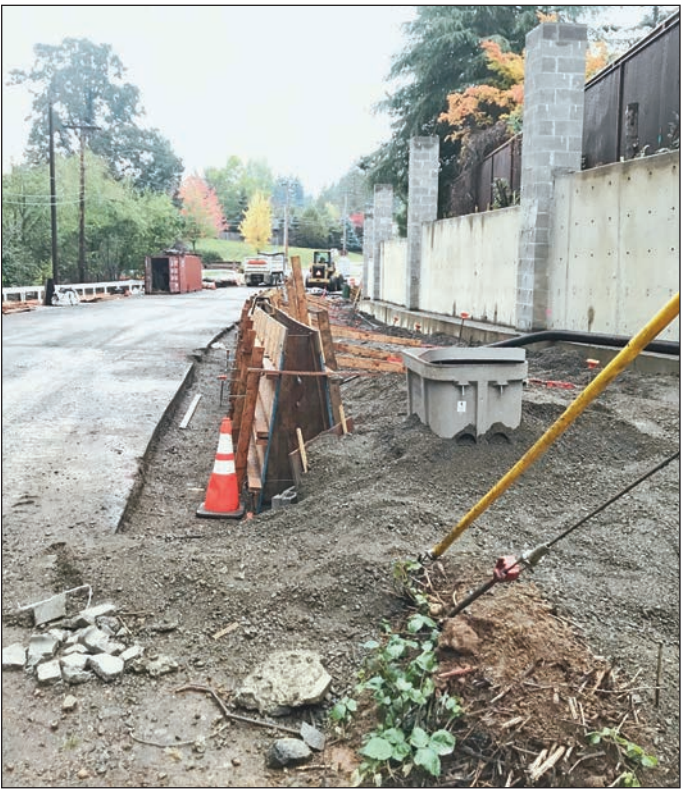
Corresponding photo shows the northern end of SE 129th Ave. Once completed, an elevated multi-use pathway will run parallel to major road improvements, allowing for safer mobility of pedestrians and bicyclists. The road previously possessed limited visibility for all modes of transport and lacked roadway shoulders.
