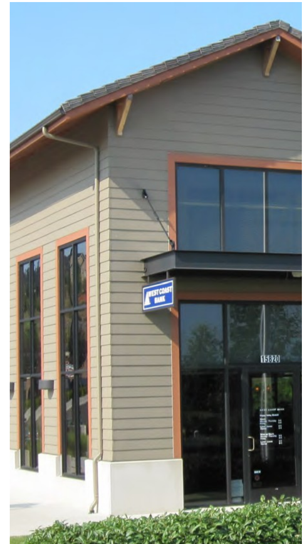
This local bank building employs traditional lap siding as primary material, which in conjunction with the gabled roof evokes a residential character. The large windows and the use of steel for window and door frames and awnings provide a contemporary contrast.
