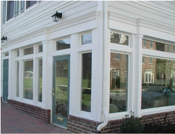
This wooden storefront evokes a residential character through scale and detailing.
