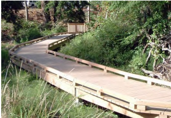
This boardwalk provides pedestrian access across a wetlands area in Woodinville, Washington.
