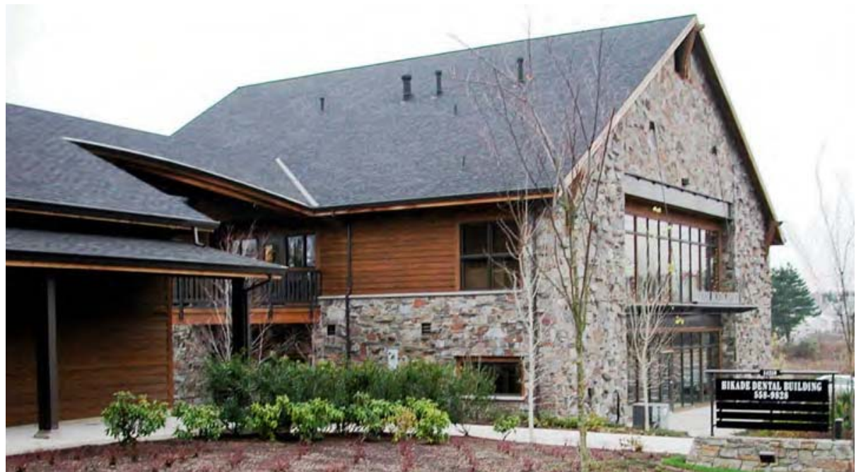
The pitched, gabled roof, asymmetry, multiple scales and varied materials of the Hikade Building (Clackamas County) contribute to its residential character.
