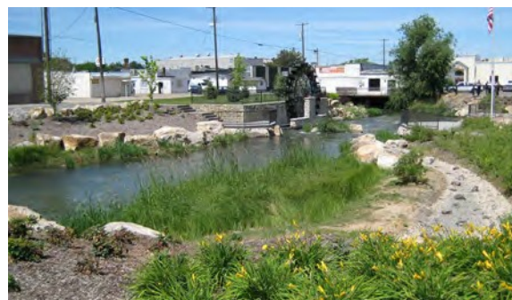
The City of Caldwell, Idaho daylighted and restored the previously buried Indian Creek through the city center to provide a public amenity and encourage development to embrace the creek.
