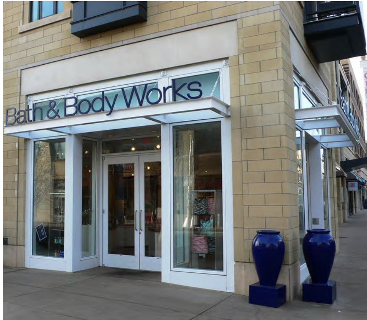
This storefront building in Denver, Colorado combines contemporary materials and detailing with proportions that evoke traditional storefronts and small town character.
