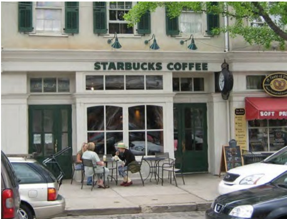
This traditional wooden storefront in the outskirts of Philadelphia, Pennsylvania complements the small town character of its surroundings.
