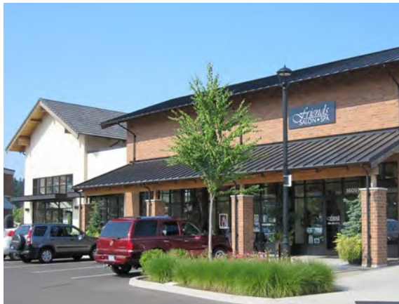
This storefront building in Happy Valley faces a sidewalk in a commercial development. The gallery provides shelter and adds visual interest.
