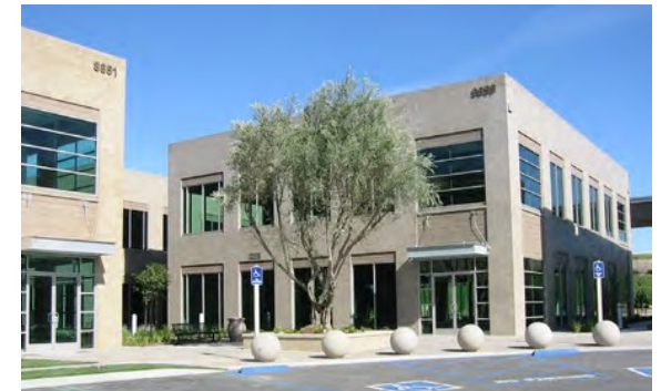
This office park development in California employs contemporary architecture and materials, however, the scale and facade patterning provides a human scaled and pedestrian friendly environment.
