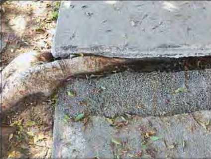
Watch out! Sidewalk concrete that has become disjointed, cracked, broken and uneven is a hazard. In Happy Valley, property owners are responsible for ensuring sidewalks adjacent to their homes and businesses remain in good working condition.
