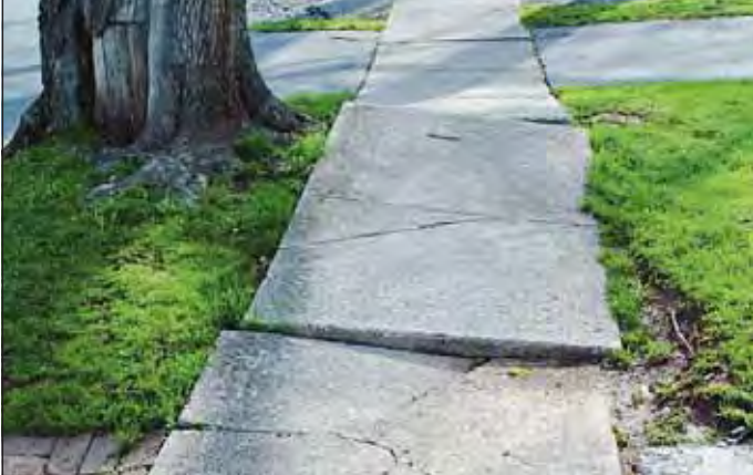
Watch out! Sidewalk concrete that has become disjointed, cracked, broken and uneven is a hazard. In Happy Valley, property owners are responsible for ensuring sidewalks adjacent to their homes and businesses remain in good working condition.
