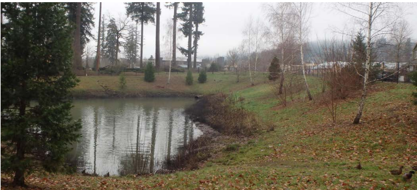
Figure 25. Example of Regional Stormwater Facility
