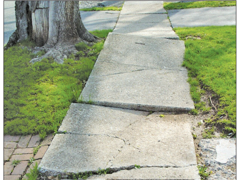
Sidewalk concrete that has become disjointed, cracked, broken and uneven is a hazard.
