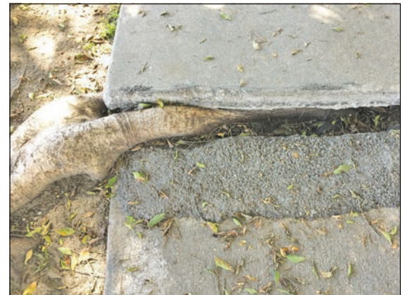
◀ Tree roots can sometimes cause concrete to lift and break.
