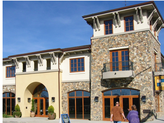
This building has a formalized tower element at the street corner. The tower is a full story taller than the remainder of the building and its facade slightly extends beyond the adjacent building facades to further accentuate the corner.
