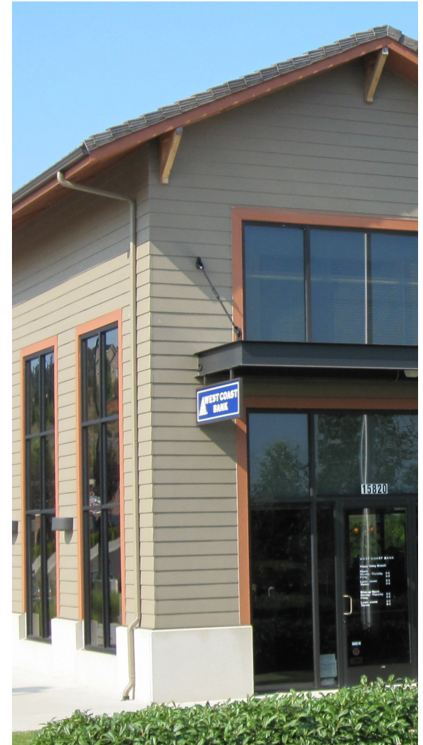
This local bank building employs traditional lap siding as primary material, which in conjunction with the gabled roof evokes a residential character. The large windows and the use of steel for window and door frames and awnings provide a contemporary contrast.
