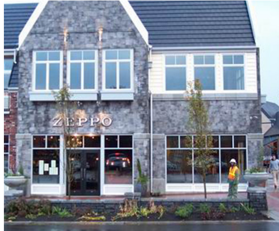
Lakeview Village (Lake Oswego, Oregon) uses rusticated stone as the primary building material for this portion of the office retail development.
