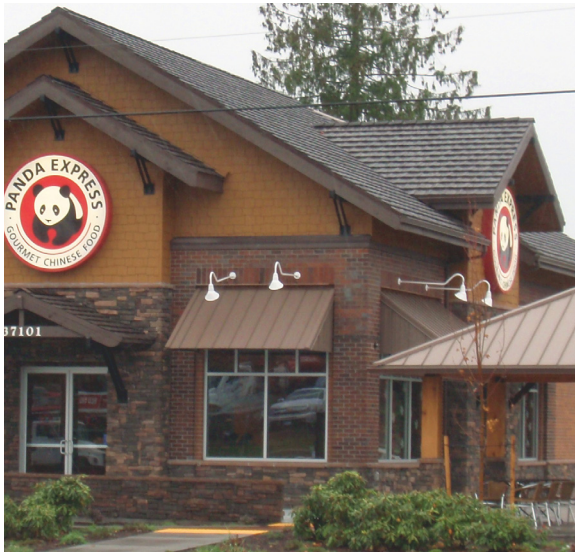
The base of this building is clad in multi-colored brick, which provides a nice contrast to the wood cladding above.
