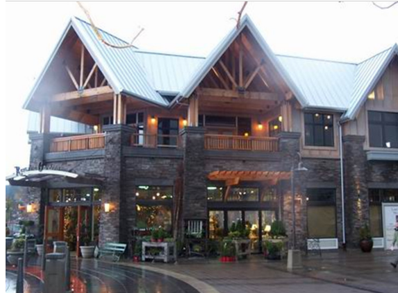
The Lakeview Village development (Lake Oswego, Oregon) is an example of a large-scale retail project that incorporates a varied roofline using steeply-pitched front gables.
