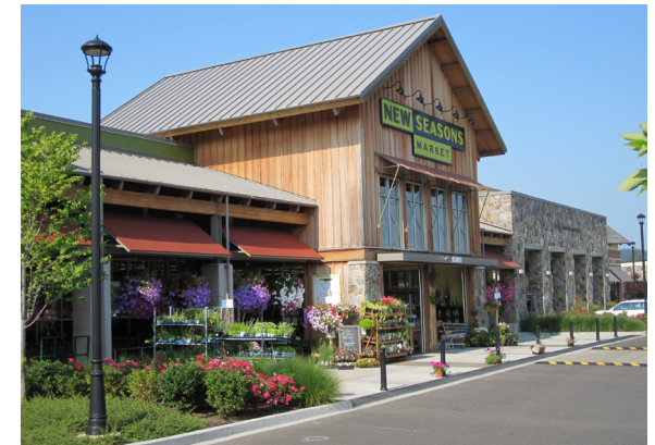
The main entrance into this grocery store in Happy Valley is quite dramatically emphasized through a central architectural element that projects out from the remaining building facade and has a steeply pitched roof.
