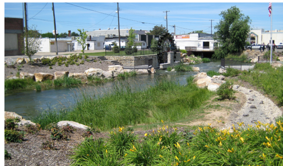
The City of Caldwell, Idaho daylighted and restored the previously buried Indian Creek through the city center to provide a public amenity and encourage development to embrace the creek.
