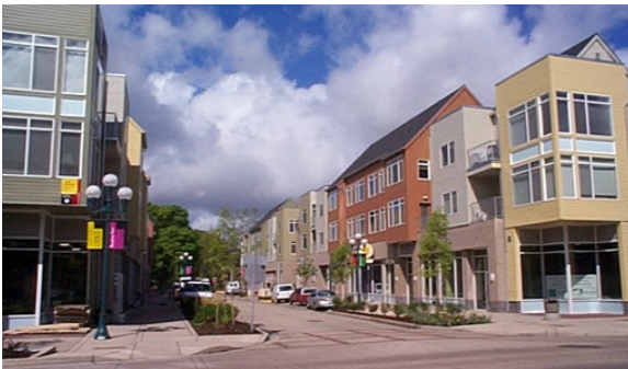
This mixed-use project in Eugene, Oregon has retail uses on the ground floor and residential above. The development incorporates characteristics of the Happy Valley Style such as varied rooflines, complex massing, strong corners and façade articulation.
