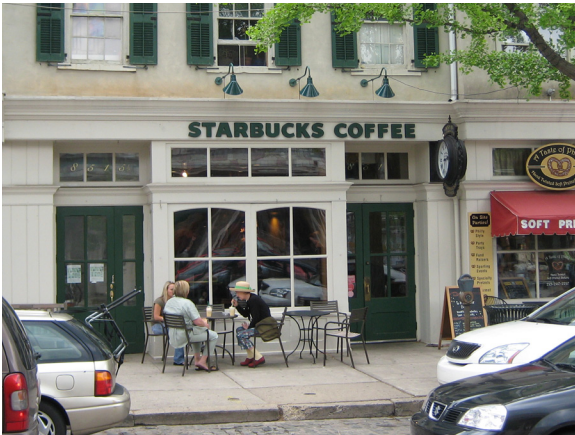
This traditional wooden storefront in the outskirts of Philadelphia, Pennsylvania complements the small town character of its surroundings.
