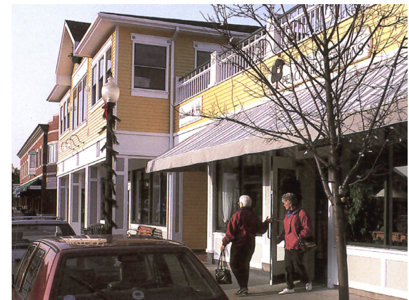
The corner emphasis in this mixed-use building is achieved through a change in both the roofline and the facade plane. The building projects above the sidewalk at the intersection to create a strong corner. The corner portion is also taller than the rest of the building.
