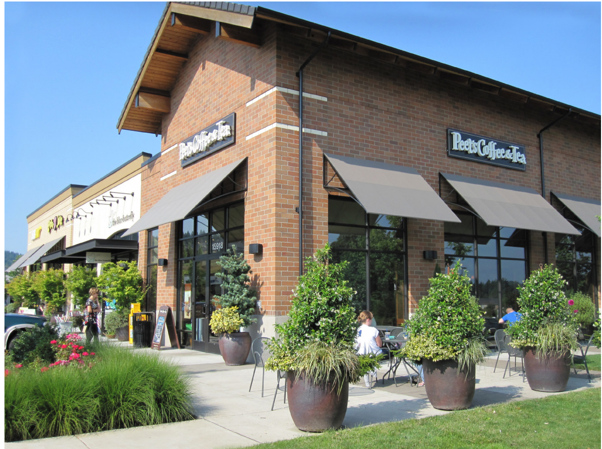
The corner building of this multi-tenant development is clad in brick and provides a contrast to the stuccoed facades.
