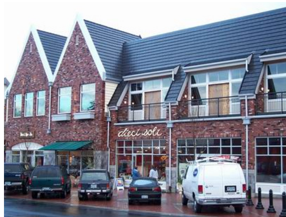
This mixed-use building in Lakeview Village (Lake Oswego, Oregon) uses ground floor windows and divided bays to create an articulated storefront appearance.
