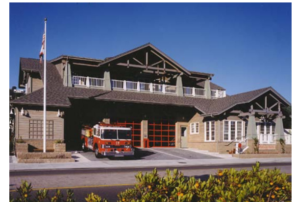
This Fire Station (Jackson, Wyoming) uses a dormer with a gabled detail and smaller front gables to achieve a varied roofline.
