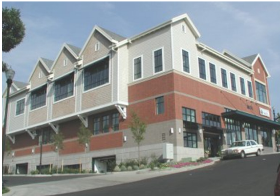
This mixed use development (Lake Oswego, Oregon) incorporates the site’s existing slope and uses it to provide below-grade residential parking and create a more compact development.
