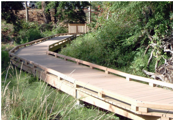
This boardwalk provides pedestrian access across a wetlands area in Woodinville, Washington.
