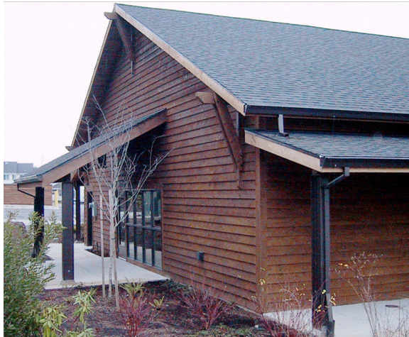
The Hikade building incorporates a variety of materials that exemplify the Happy Valley Style, including stone (primary material), wood, glass and steel. The building's side wing is clad in wooden lap siding, evocative of a barn structure.
