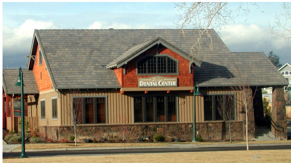
This dental office in Bend, Oregon is designed with a residential character to be compatible with the surrounding neighborhood.
