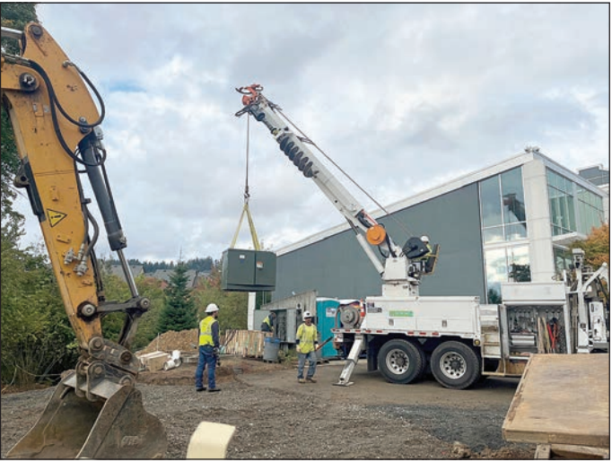
A crane lifts the generator and begins moving it to its new location.
