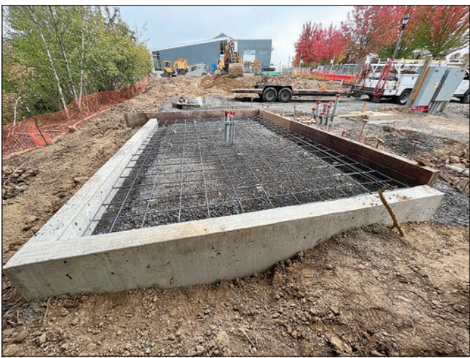
A new pad is poured for the generator and transformer.
