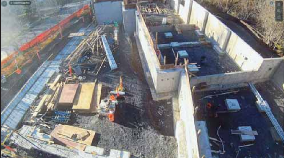
An aerial view of the construction progress shows the library expansion footings and initial wall formations.
