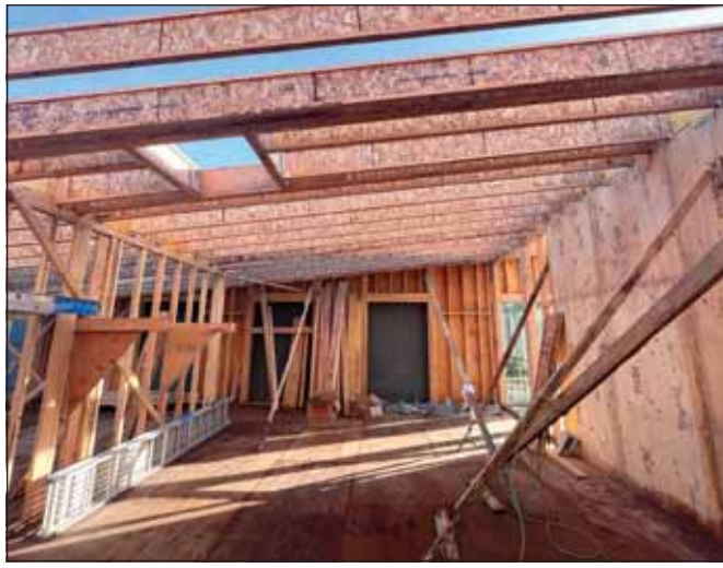
Roof joists and glulam beams were installed.
