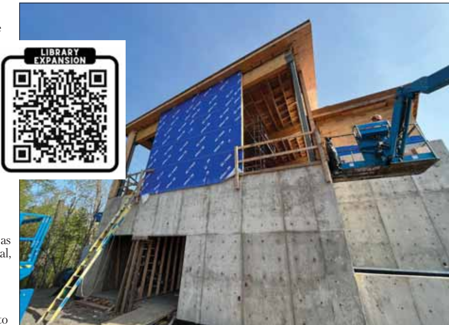
CREWS WORK TO ENCLOSE THE STRUCTURE AND PREPARE IT FOR SHEETROCK.
