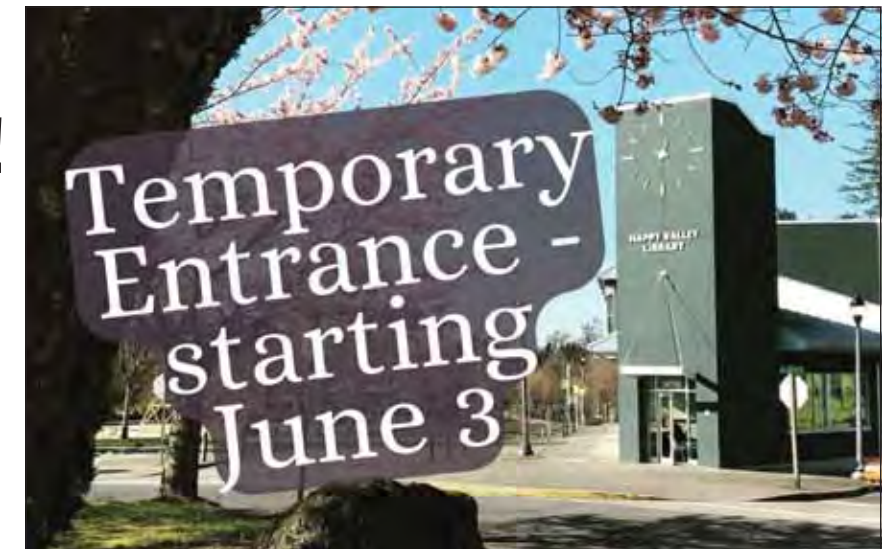
The library's main entrance to shift temporarily during the next phase of construction.
