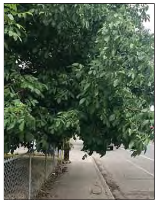
Tree branches and shrubs that encroach in the public right-of-way can create a safety hazard. Ensure your sidewalks and streets remain clear for travel so pedestrians and service vehicles can pass easily. PHOTO COURTESY OF CITY OF HAPPY VALLEY
