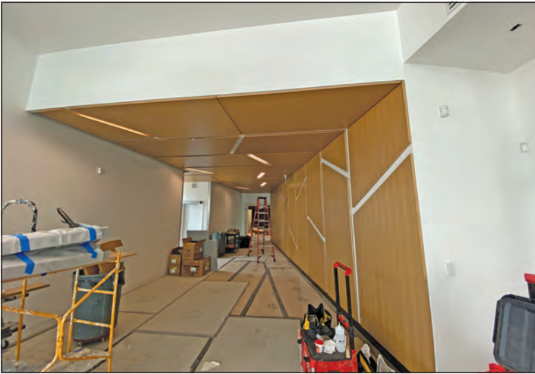
PHOTO COURTESY OF CITY OF HAPPY VALLEY Acoustical panels being installed in the lobby.
