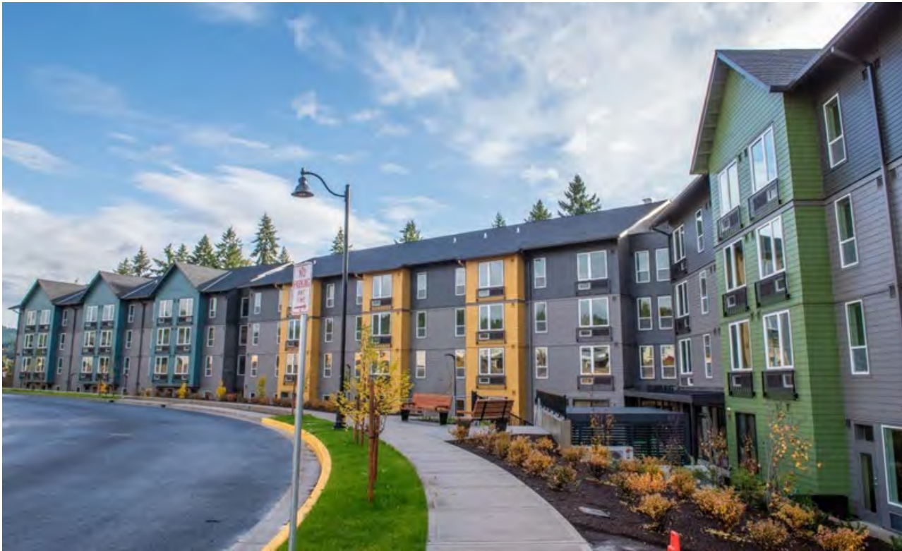
Figure 4-7. Good Shepherd Village, Affordable Housing in Happy Valley (Image credit: Catholic Charities)
