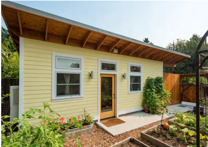
Figure 4-8. A No-step Entry Backyard Accessory Dwelling Unit (ADU) (Image credit: SQFT Studios)
