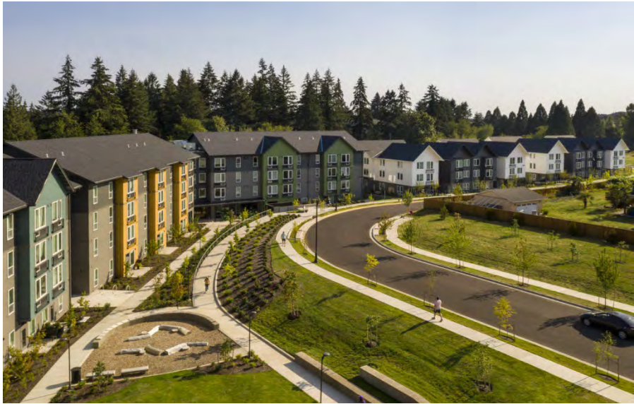
Figure 4-9. Right-of-way Improvements for Affordable Housing Development in Happy Valley (Image credit: MWA Architects)
