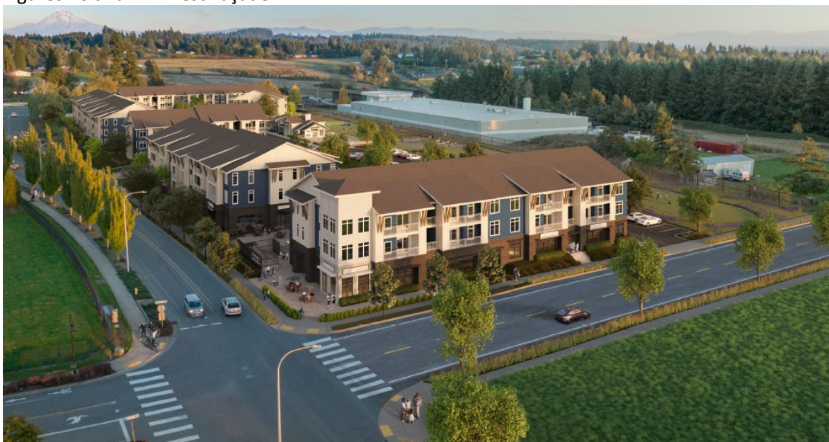
Figures 10 and 11: West Façade
