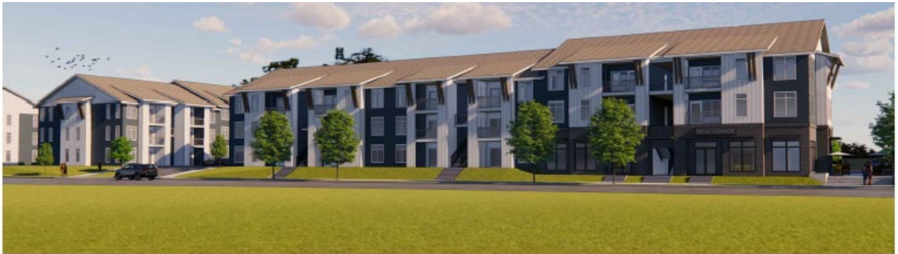
3 BUILDINGS 2 & 3 - VIEWING FROM ROCK CREEK BLVD
