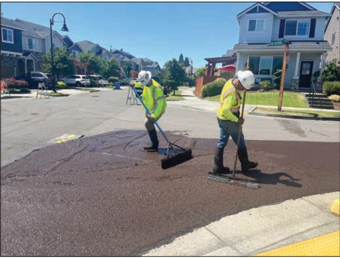
Slurry seal treatment is spread on the top of roadways to help extend their life.
