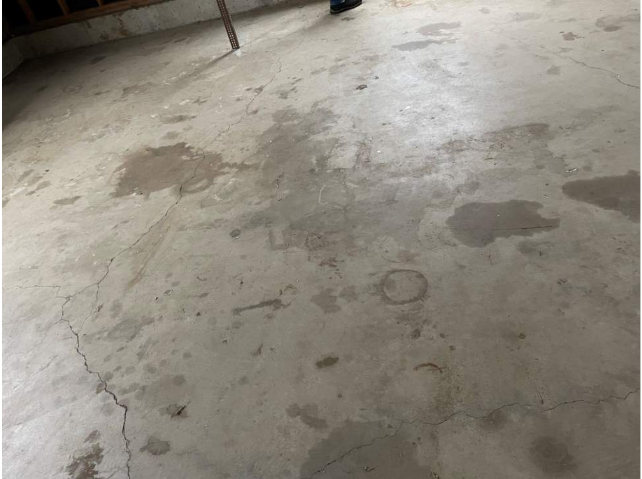
Staining on the concrete in the garage
