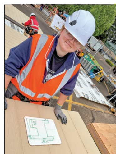
A student from the advanced construction class of Sabin Schellenberg Professional Technical Center works on the side of a shed they built for the Construction Industry Education Foundation Design Build Competition.
