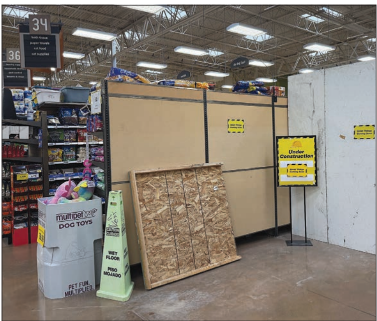
The remodel project at the Happy Valley Fred Meyer continues.
