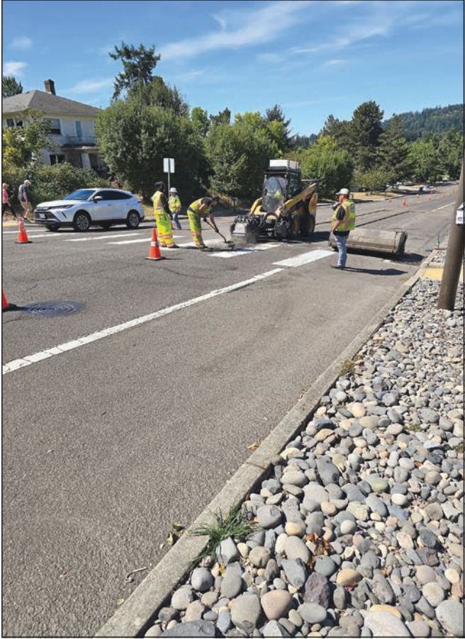
Road crews repaired a pot hole along King Road.
