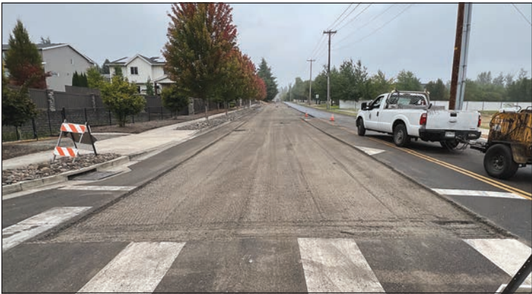
As part of the City's ongoing commitment to accessibility, crews upgraded 29 curb ramps this year.
